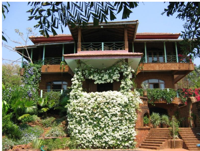
The Tree House, designed and landscaped by John Hicks
